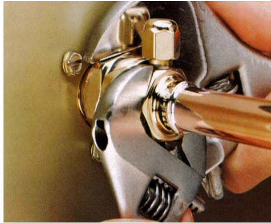
Use Two Wrenches to Tighten
